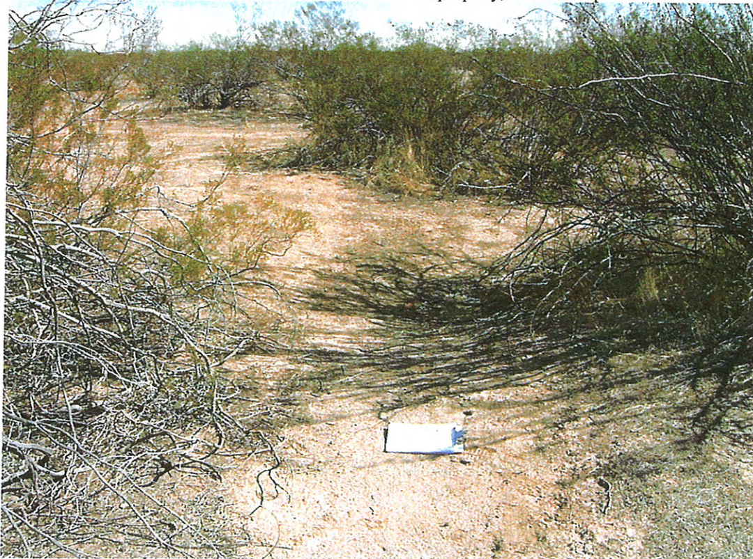
Figure 7: Resulting offsite dispersion and dissipation of flows from the culvert in Figure 6.
