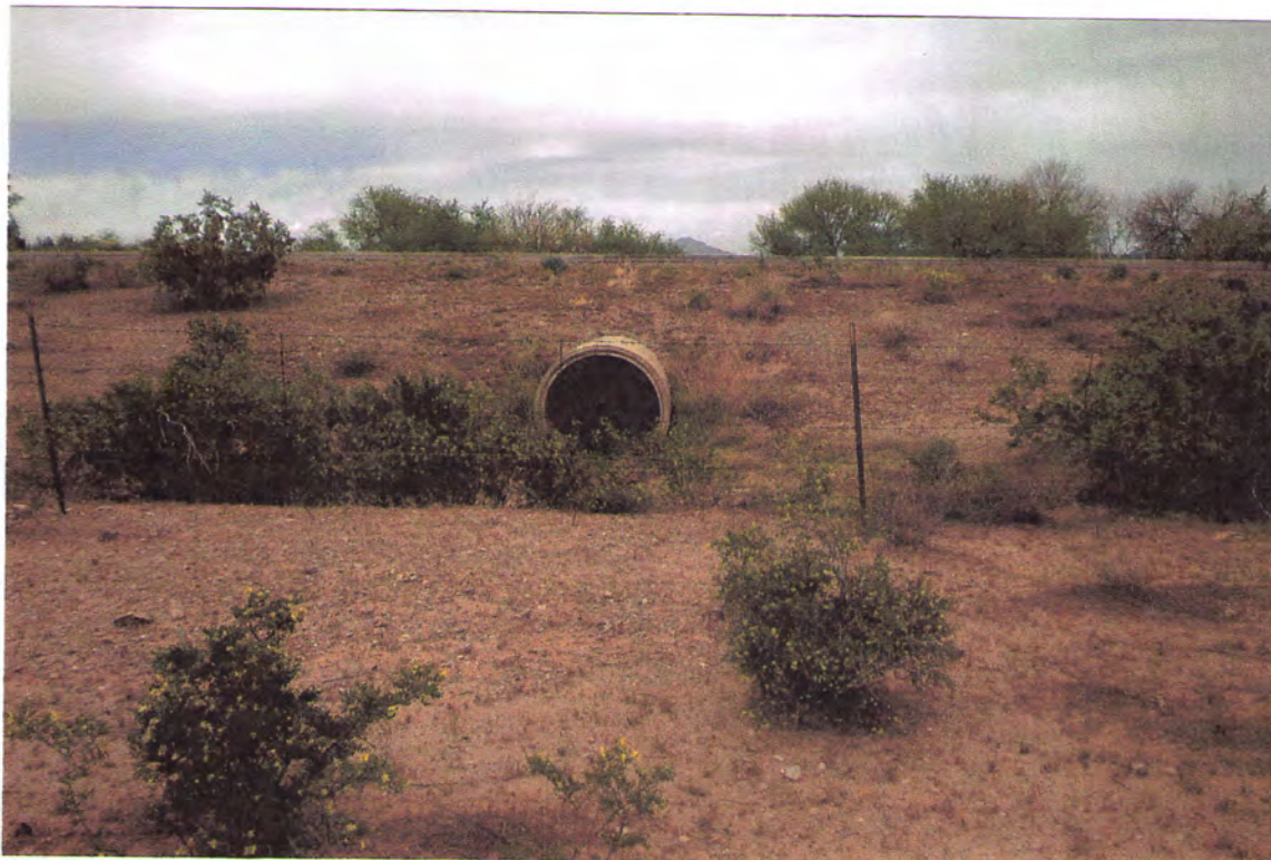
Photograph #20 - View of storm drain entering south parcels from north vicinity -
