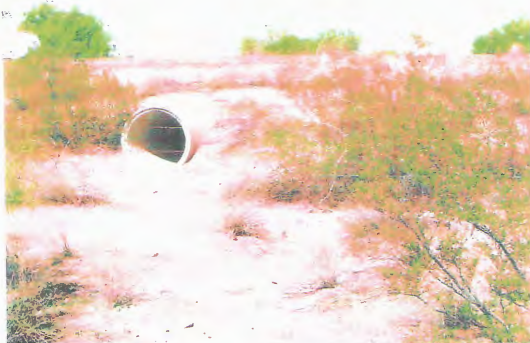
Figure 6: A culvert seen from the extreme northwest portion of the Parcel. Flows from the northern slopes of the Parcel are channeled here and other culverts under I-8 off property, which dissipate to sheet flow.
